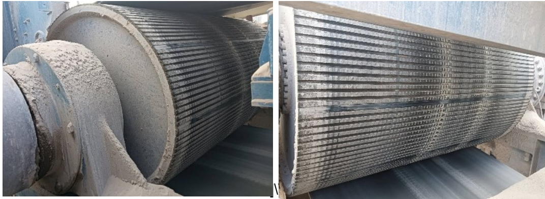
Figure 3: Conveyor drive pulley item no. 2 in Table no.1
